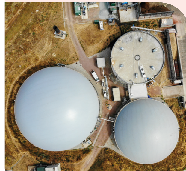
Grange Farm anaerobic digestion plant, Lincolnshire, UK
