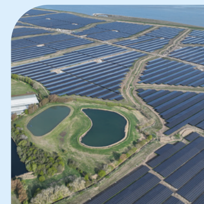
Quinbrook's Cleve Hill Solar Park in Kent
